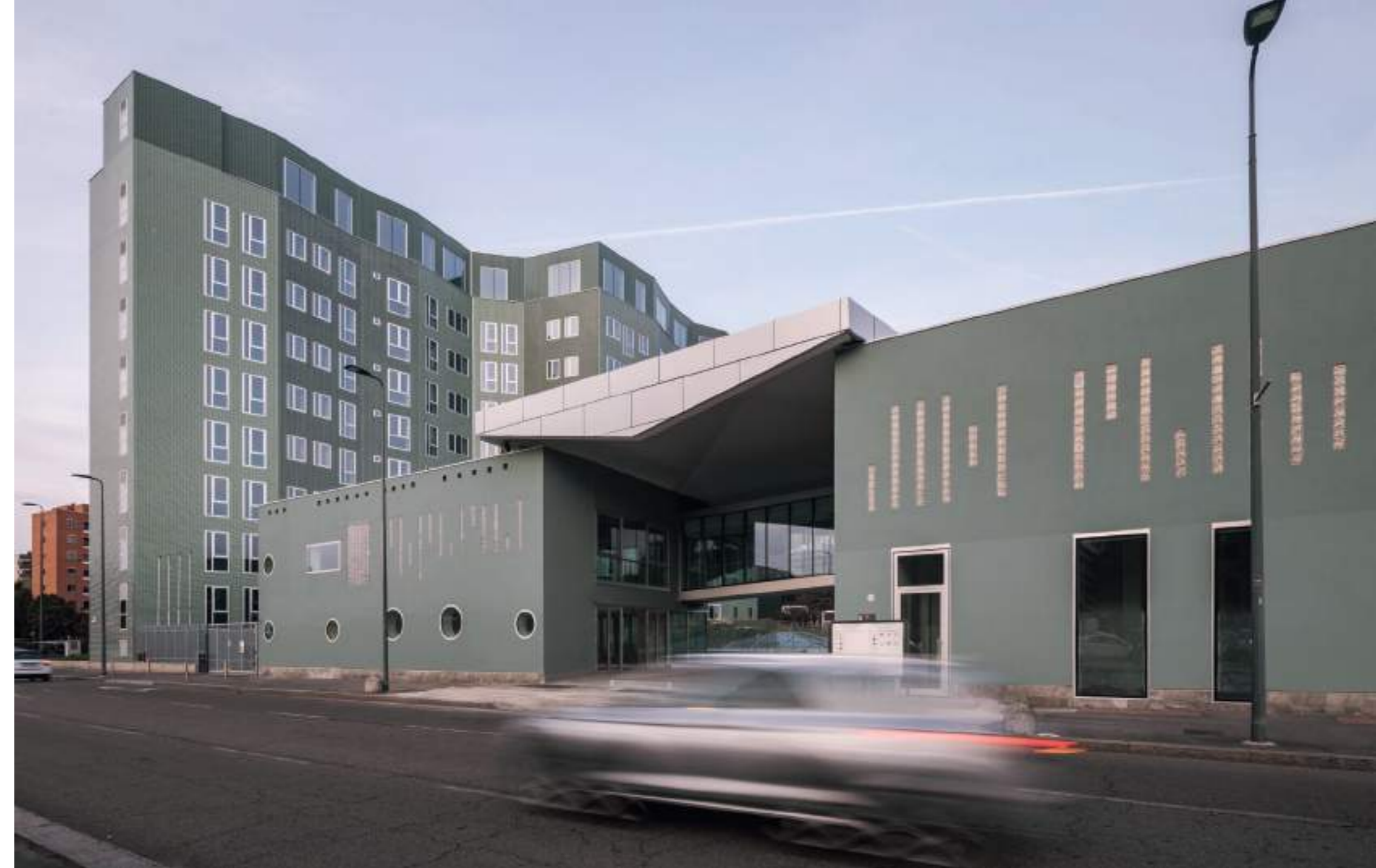
VISTA DA VIA SAN VIGILIO VIEW FROM VIA SAN VIGILIO
